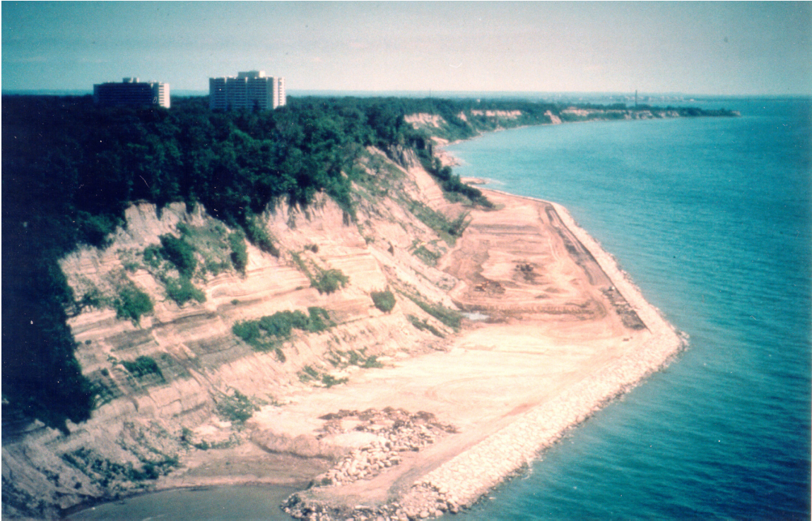
Figure III-5-24. Shore protection consisting of a wide berm protected by a revetment along the base of the Scarborough Bluffs located east of Toronto on Lake Ontario
